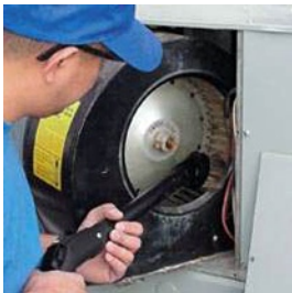
Cleaning ventilation blower blades.
