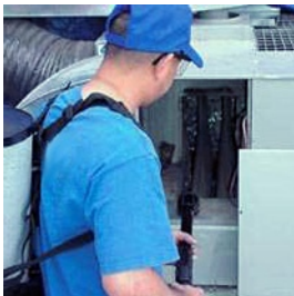
Cleaning the air conditioning unit.
