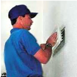
Remove vents, registers and diffusers.
